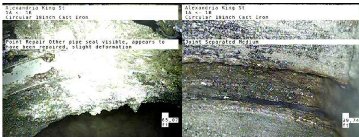
Point repair of pipe crown but has slight deformation
