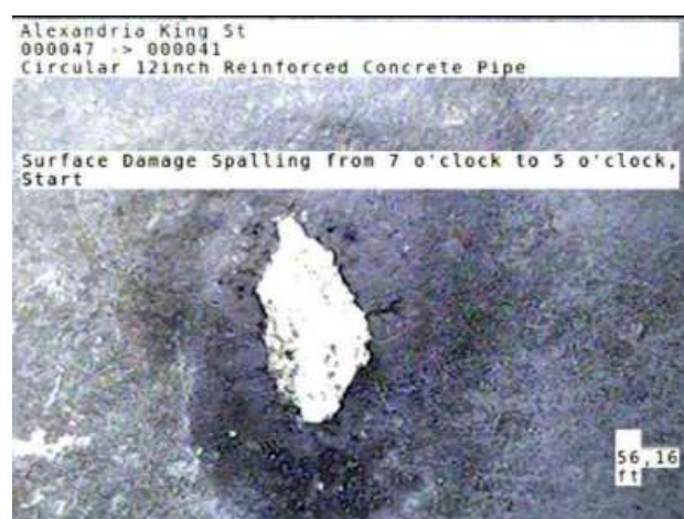
Spalling damage of pipe surface
