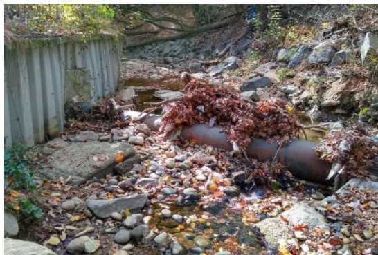
Exposed sanitary pipe adjacent to a deteriorating sheet pile wall (left), with a riprap-lined channel bank providing erosion control on the right.
