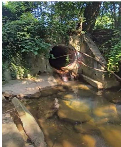
Deteriorating outfall and concrete debris in plunge pool
